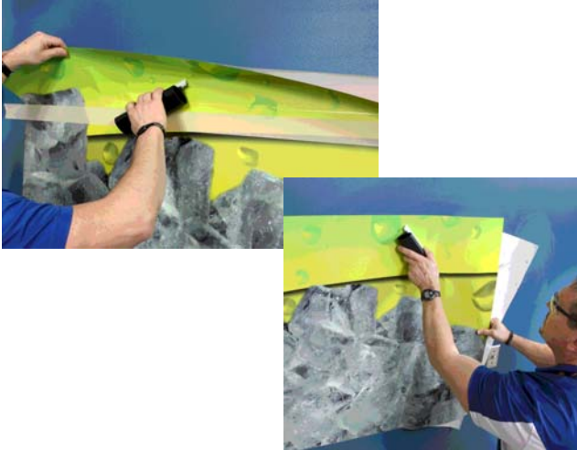
FIGURE 17 Keep Tension on the Unapplied Film
