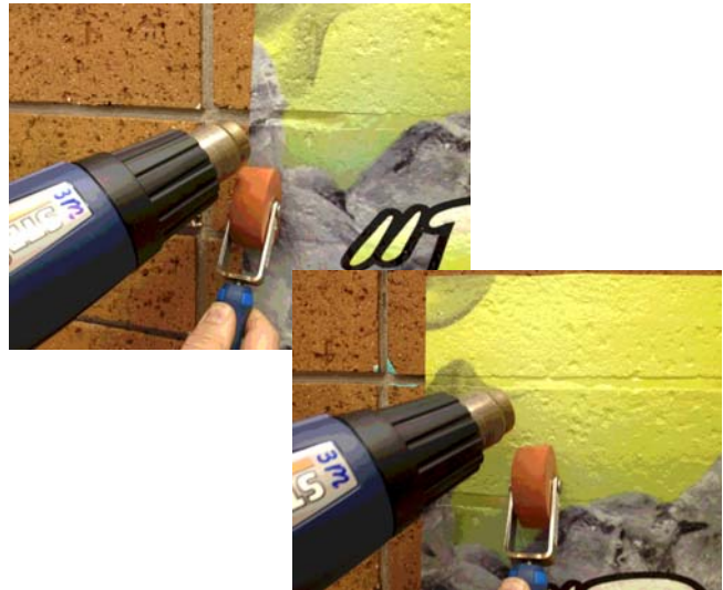
FIGURE 32 Use the TSA-3 Tool and Heat Gun to Touch Up Poorly Adhered Areas
