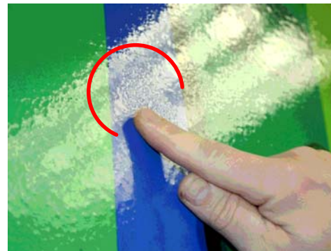
FIGURE 19 Check for Full Adhesive Contact with Wall
