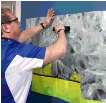
FIGURE 14 Squeegeeing Exposed Adhesive for Self Hinge
