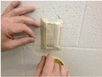
FIGURE 35 Cover the Obstruction with Masking Tape
