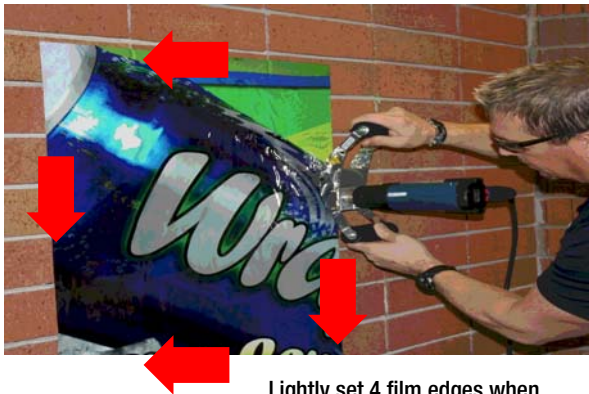
Lightly set 4 film edges when applying to deep grout lines, if desired
