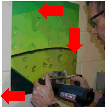
FIGURE 28 Lightly Set 3 Film Edges
